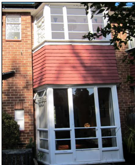
Original rear elevation (inc. toilet and larder windows)
