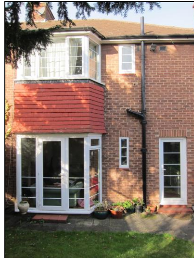
Reproduction rear elevation (inc. toilet and larder windows) (with 25mm internal 'Georgian' bars)
