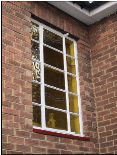
Original landing window
