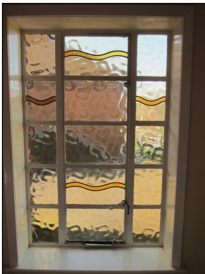
Original landing window (internal view)
